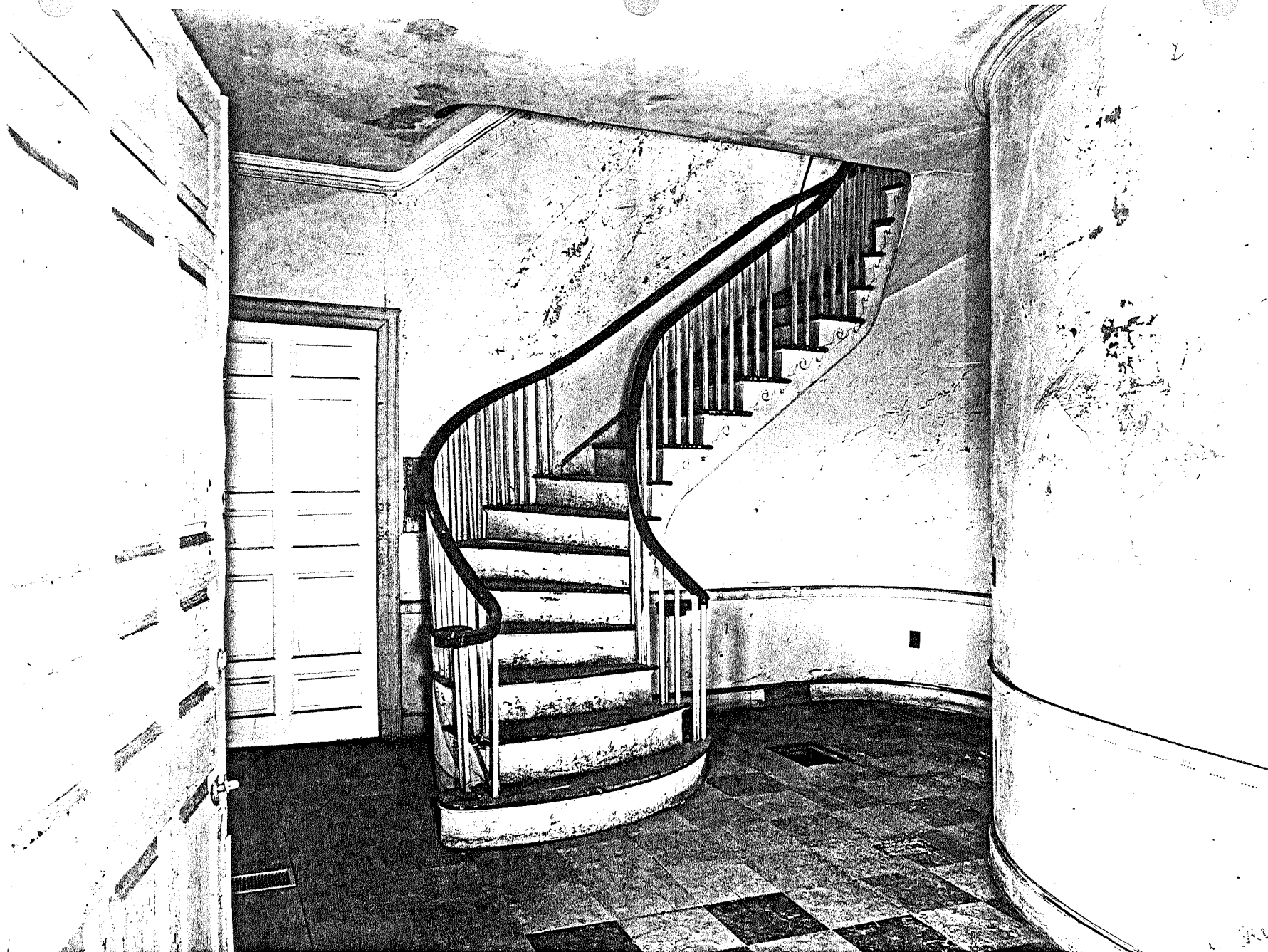
Fig. E-6. Shirley-Eustis House, Roxbury, Ma. West vestibule looking north showing Georgian period floor, doors, and evidence of former partitions in ceiling; Federal period stair, dado, and plaster patches and cornice; Modern paint. J. David Bohl photo, August, 1979. (SPNEA)
