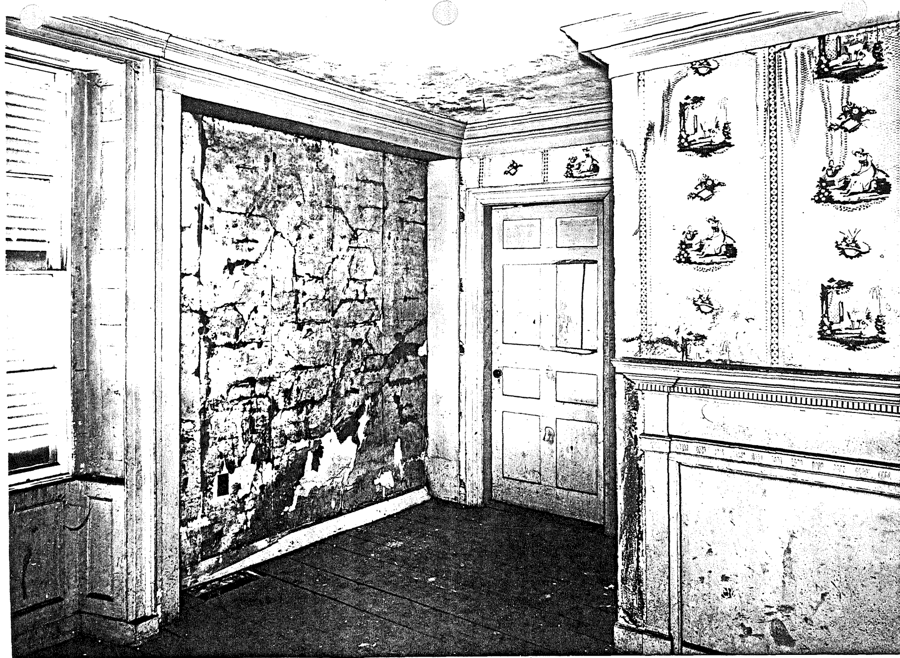
Fig. E-19. Shirley-Eustis House, Roxbury, Ma. Northwest Library chamber looking northeast showing Georgian floor, alcove, cornice at left, and door; Federal window and door trim; Victorian porcelain "mineral" door knob; Modern chimney breast restoration at right with salvaged Federal mantel of unknown origin, Modern cornice and wallpaper. J. David Bohl photo, August, 1979. (SPNEA)
