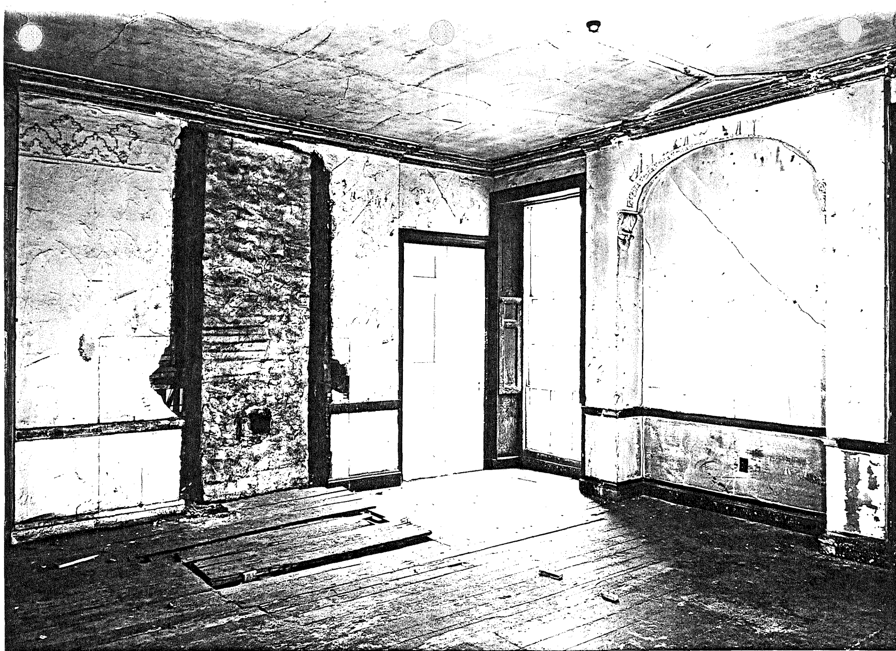
Fig. E-16. Shirley-Eustis House, Roxbury, Ma. Northeast Dining Room looking northwest showing Federal painted walls with silhouette of former mantel shelf, floor, ceiling, ornamental plaster cornice, sideboard alcove, window, false double door and trim; Victorian fireplace alterations, partition evidence, and wallpaper under Modern paint. J. David Bohl photo, August, 1979. (SPNEA)
