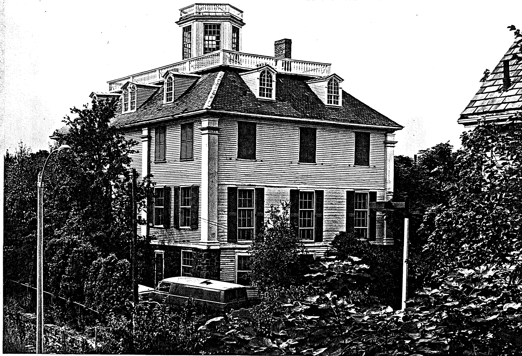
Fig. E-3. Shirley-Eustis House, Roxbury, Ma. Northeast view showing Georgian pilasters, balustrade, and cupola sash; Federal siding, windows, sash, blinds, dormers and cupola balustrade; Victorian foundation, chimney, slate roof and double dormer on east slope (left); Modern basement level infill north end (right). J. David Bohl photo, August, 1979. (SPNEA)
