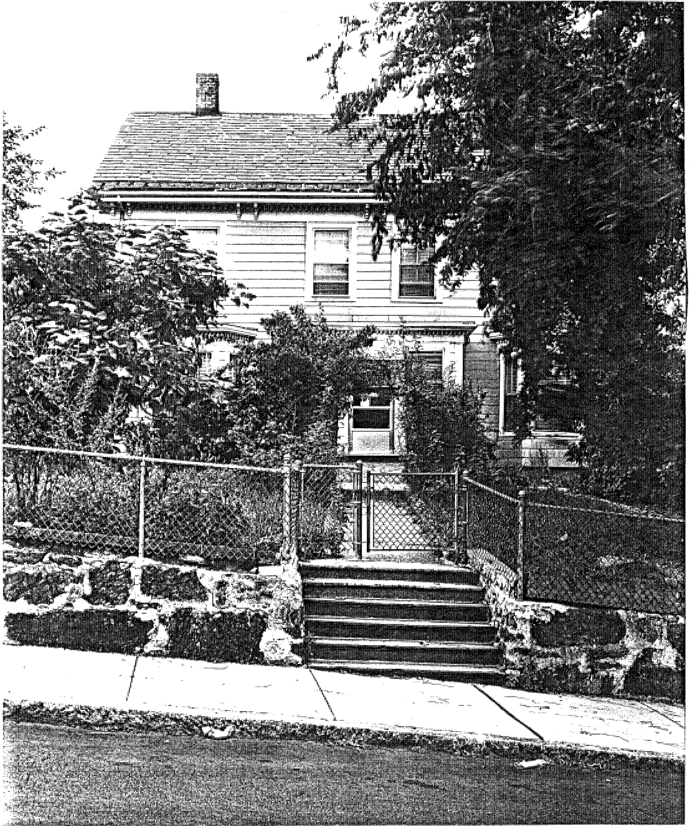
Fig. E-4. View of double house, No. 42-44 Shirley Street, traditionally part of original Shirley-Eustis Barn. Note brownstone steps with molded nosing similar to those shown in ca. 1867 photo of Shirley-Eustis House (Fig. C-2). J. David Bohl photo, August, 1979. (SPNEA)
