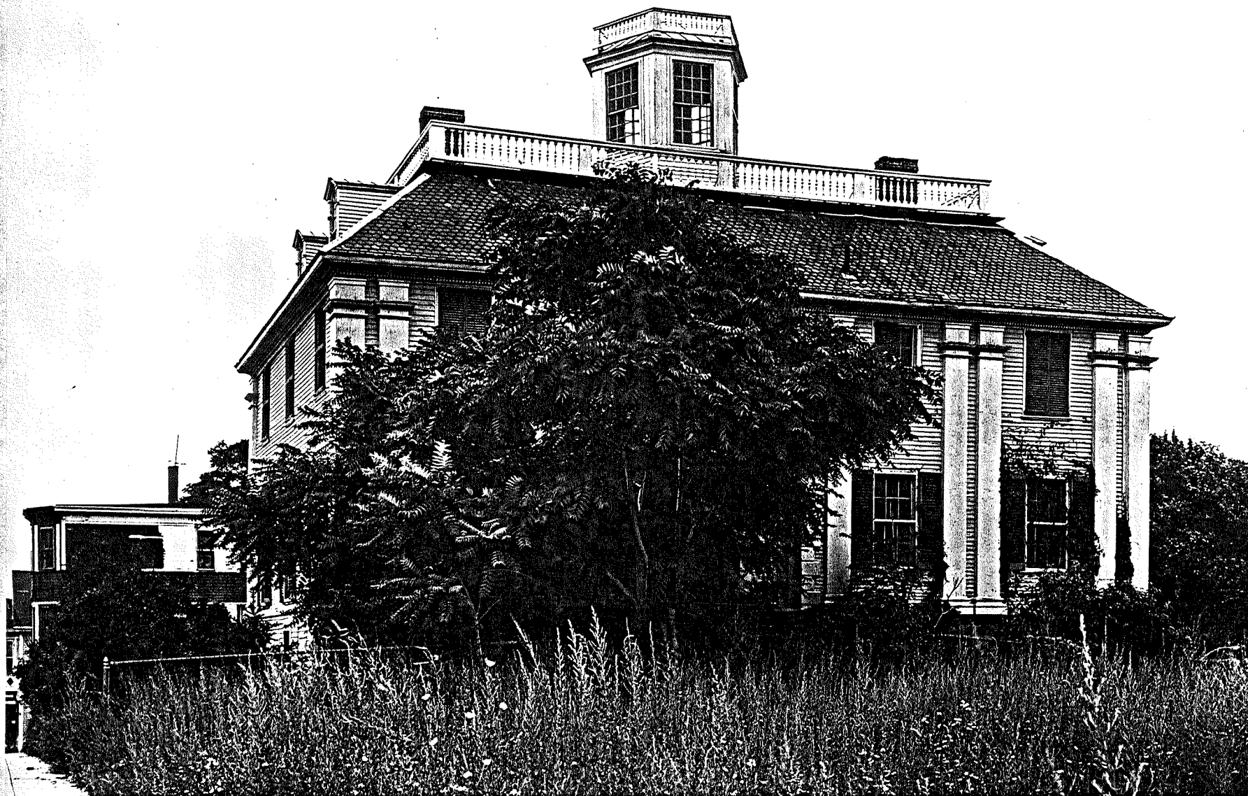
Fig. E-1. Shirley-Eustis House, Roxbury, Ma. West Front, showing overgrowth of vegetation since ca. 1970-72 restoration. Datable elements are Georgian pilasters, balustrade, cupola sash, front doorway; Federal clapboards, pilaster capitals, cornice, sash, blinds, and cupola balustrade; Victorian slate roof and chimney. J. David Bohl photo, August, 1979. (SPNEA)
