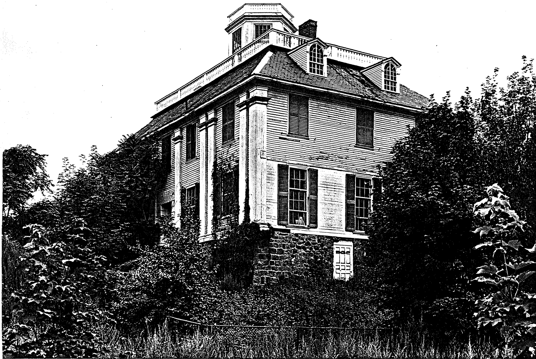
Fig. E-2. Shirley-Eustis House, Roxbury, Ma. Southwest view showing overgrowth since ca. 1970-72 restoration. Note deterioration of slate roof, water table, corner pilasters. Datable elements are Georgian pilasters and balustrade; Federal siding, pilaster capitals, cornice, dormers, window sash and blinds; Victorian foundation and chimney; Modern restored basement door. J. David Bohl photo, August, 1979. (SPNEA)
