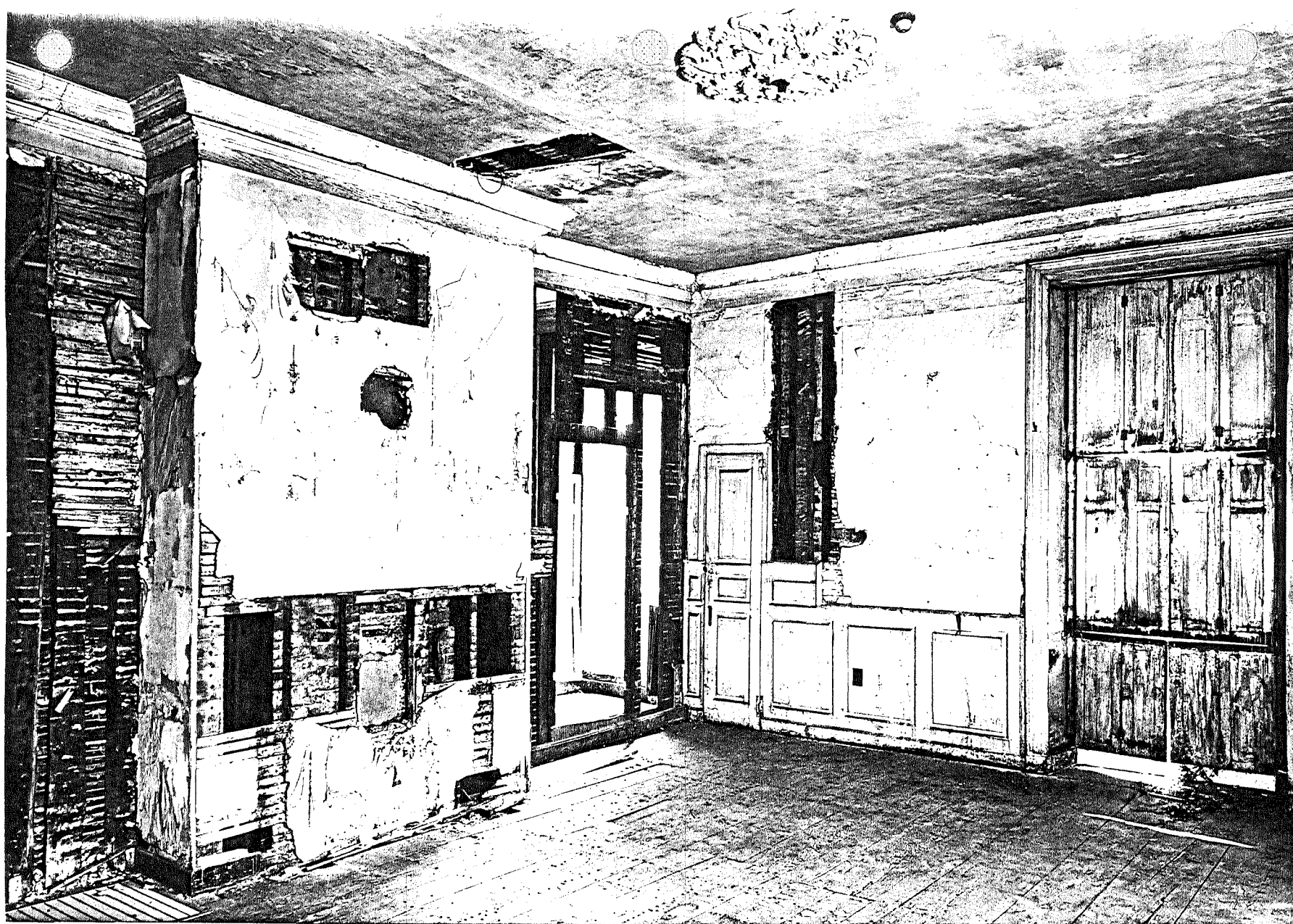
Fig. E-8. Shirley-Eustis House, Roxbury, Ma. Southwest Breakfast Room looking southeast showing Georgian dado, closet door, wood cornice; Federal window shutters, partition evidence and plaster patch above dado; Victorian floor and ceiling patches, plaster cornice, ceiling medallion, relocated door opening to drawing room. J. David Bohl photo, August, 1979. (SPNEA)
